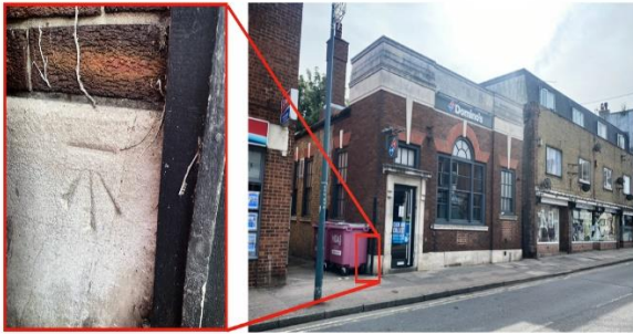
A Benchmark in Station Road
