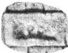
Close-up of brick showing "PC" clearly embossed in the frog
