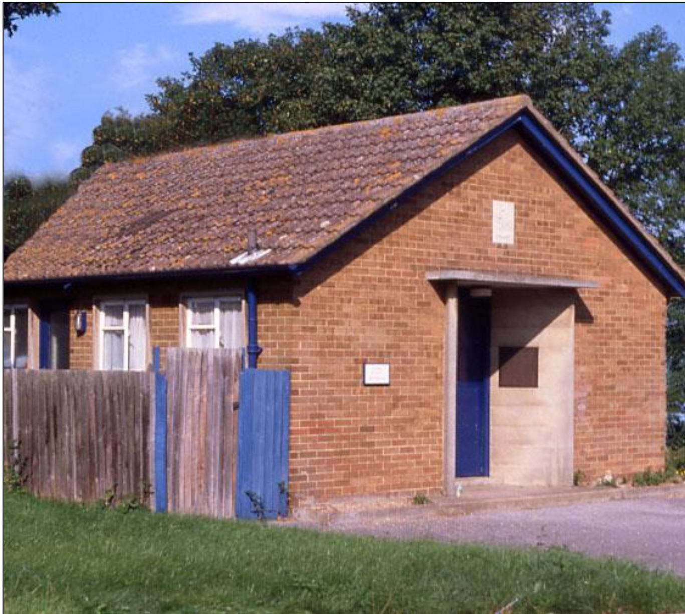
The Police sub station was built at the entrance to Birchington railway station in the early 1960s. It was built to replace the blue Police Box that had stood in the Square since the late 1930s. It was closed in the later 1960s and stood empty till the Masonic Lodge bought it.
