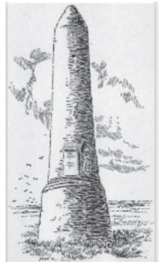
By the late 19<sup>th</sup> and early 20<sup>th</sup> centuries the beacon was neglected as such structures became less important to shipping. In August 1920 it was inspected and found to be in poor condition, the brickwork cracked and bulging. The cost of repair would be considerable, and two years later it was Scheduled for demolition, and by 25<sup>th</sup> October 1922 it was gone.
