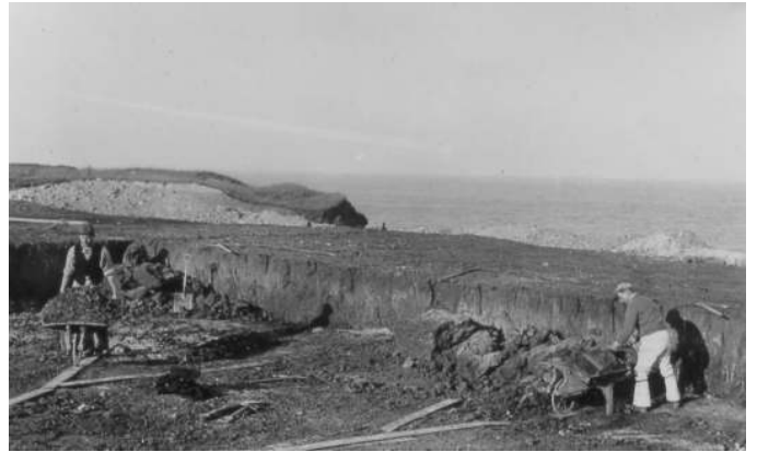
Brickfield diggers c. 1910 - At Epple Bay
